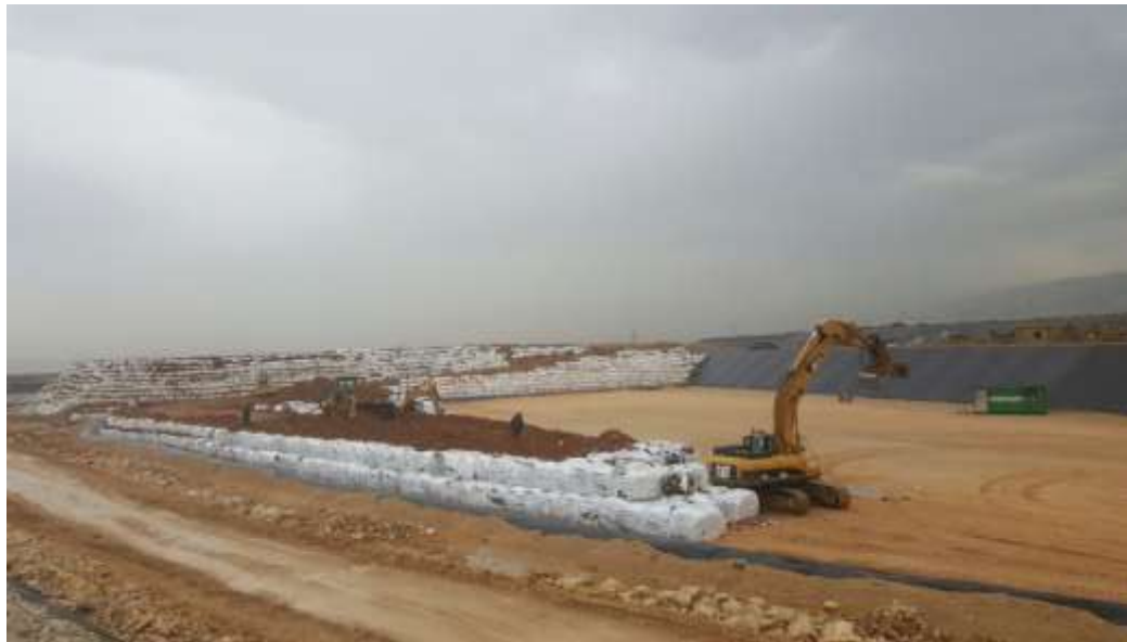
Costa Brava Sanitary Landfill
